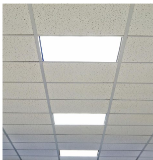
(An example of a drop ceiling)
